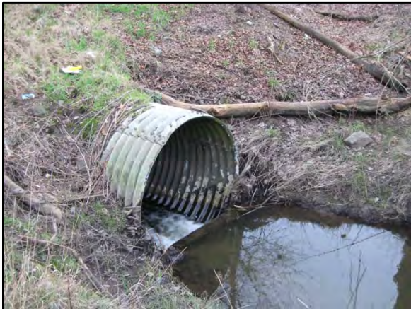
Photo 13. Gilliam Creek: view of the log at the inlet to WSDOT-owned culvert at the northbound I-405 on-ramp (fish passage ID 14611, partial barrier). (Date: 2/3/2011)
