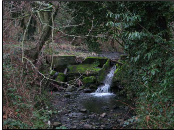
Photo 17. Upper Gilliam Creek: view upstream from the City-owned culvert under 42nd Ave S, toward the dam feature located on privately-owned property (fish passage ID 44991, total barrier). (Date: 2/4/2011)
