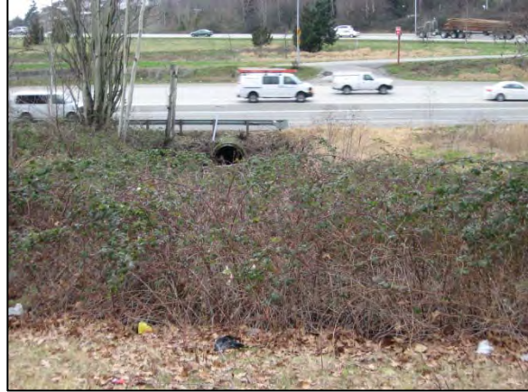
Photo 16. Gilliam Creek: view of the presumed outlet of the culvert under the I-5/I-405 interchange (fish passage ID 14737, total barrier). It was not clear from the available mapping whether this culvert conveys flow from upper Gilliam Creek, or from stormwater detention managed by WSDOT. (Date: 2/3/2011).
