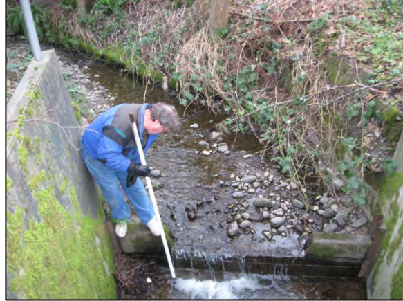
Photo 12. West Fork Southgate Creek: view of weir at the inlet to the long culvert under S 133rd Street (fish passage ID 50021, total barrier). The weir's height exceeds the fish jumping criteria by 0.10 foot, and the culvert just downstream was considered too steep for fish. Habitat just upstream provides some suitable spawning gravel, possibly for resident trout. (Date: 2/3/2011)
